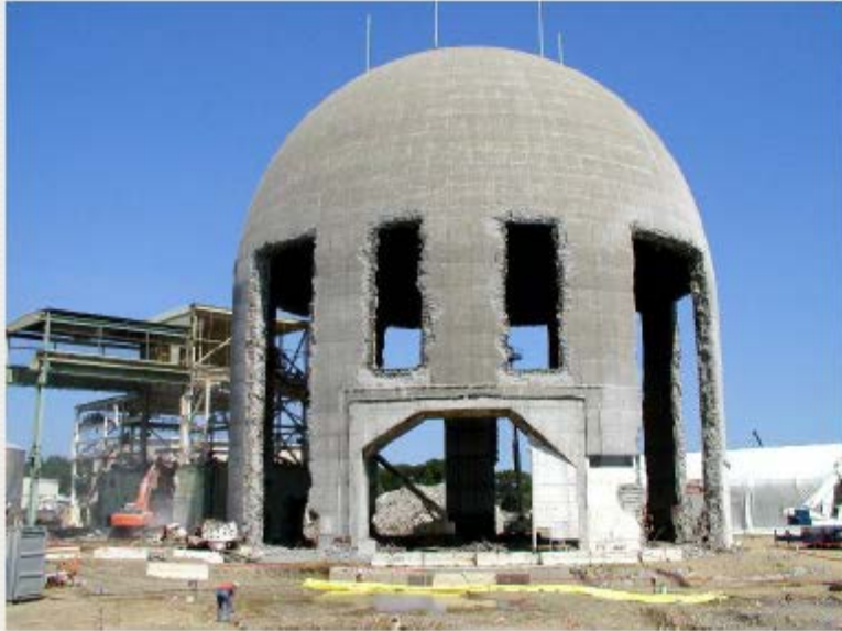
Maine Yankee being dismantled, USA
