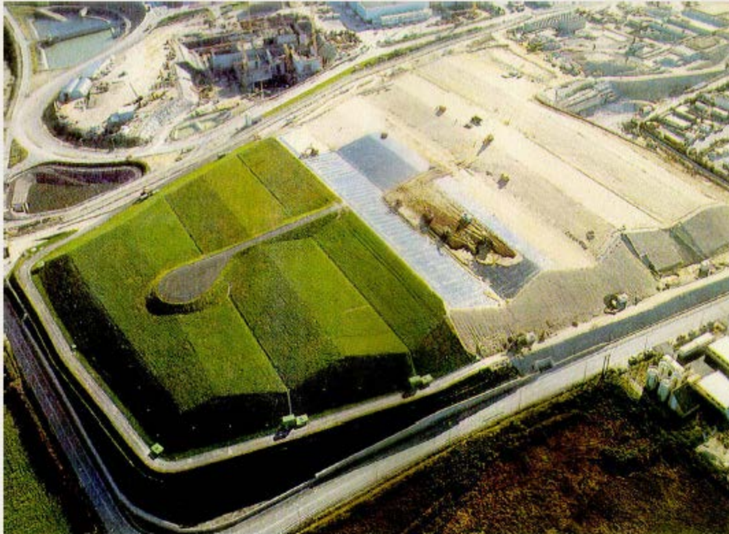
Final Covering of the Low Level Waste Disposal Facility at Centre de la Manche (France)
